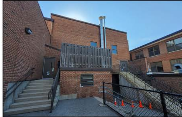
Figure 1: Outdoor utility transformer
